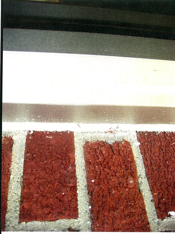
Asbestos containing door Caulking
