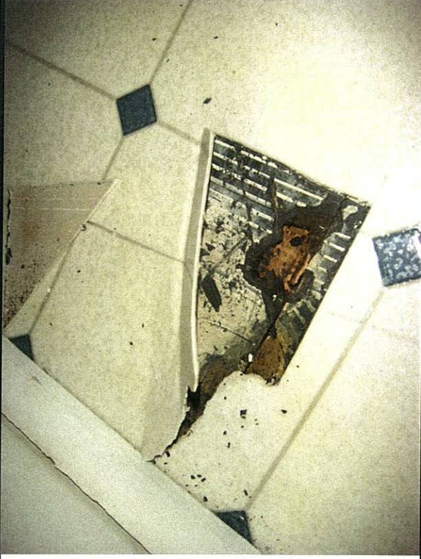
Asbestos Containing Mastic on the bottom layer of floor tile in the kitchen
