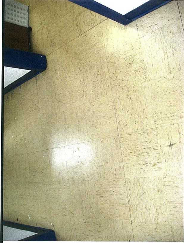
Asbestos containing 12 inch tan floor tile and floor tile mastic located under pink carpet in Hallway 1 of the BOE offices
