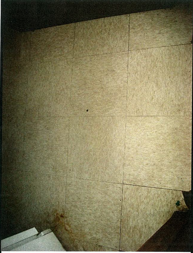
Non Asbestos Floor tile in Room 1
