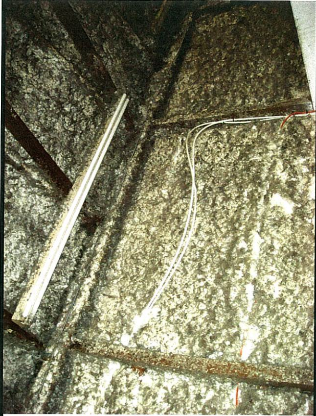
Landfill Maintenance Building Spray Applied Insulation
