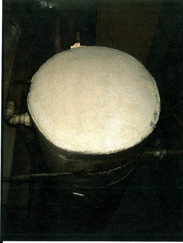
Asbestos containing insulation on the end cap of the expansion tank in the basement
