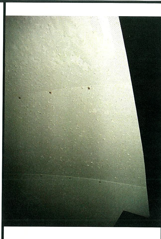
Assumed ACM Roofing material on Entire Building
