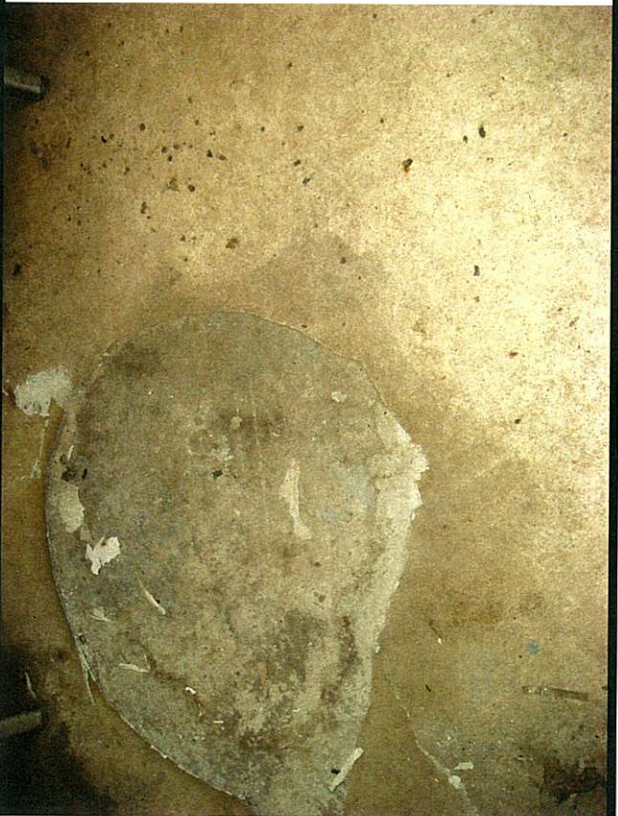
Non Asbestos Vinyl flooring in Office 1
