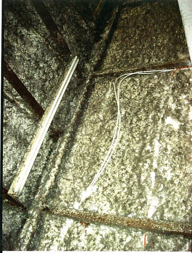
Landfill Maintenance Building Spray Applied Insulation
