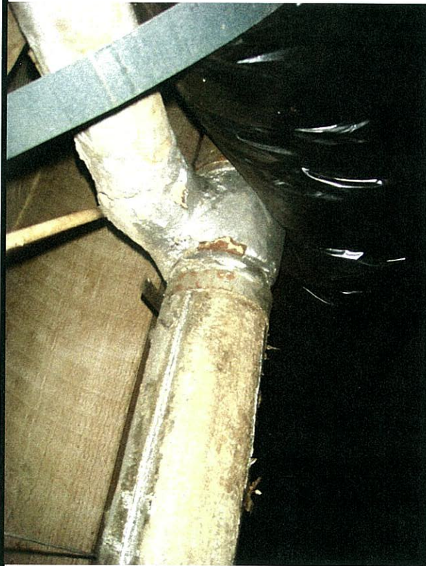
Asbestos Containing Hard elbows on hot water lines in the crawl space and basement
