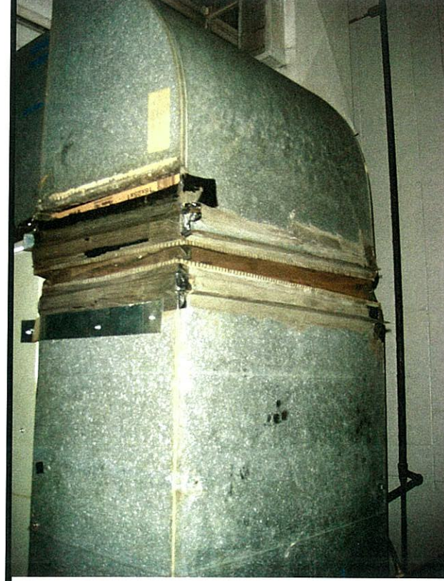
Example of Assumed Asbestos containing Vibration Damper
