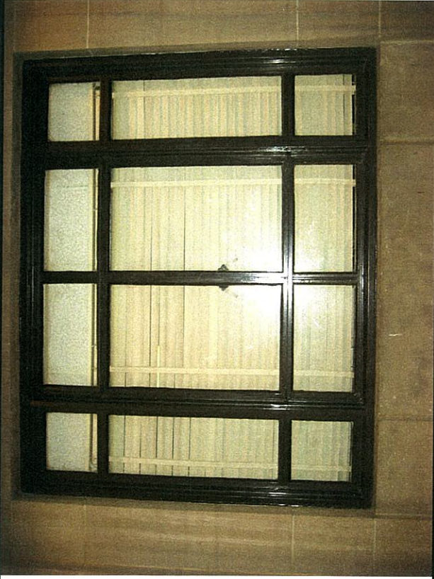
Metal Window Frames Painted Brown (LBP) and Glazing (ACM) in Main Lobby.
