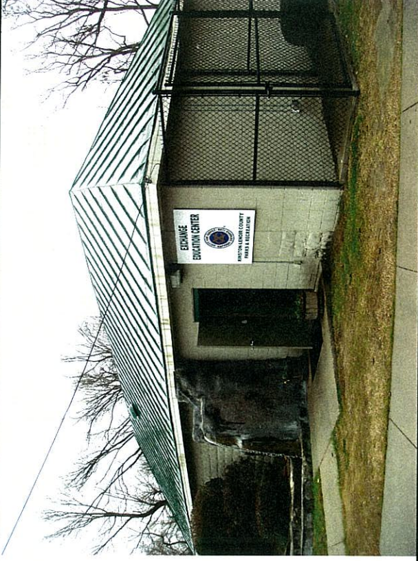
Education Building with Assumed Asbestos Containing Paint coating on metal seamed roof
