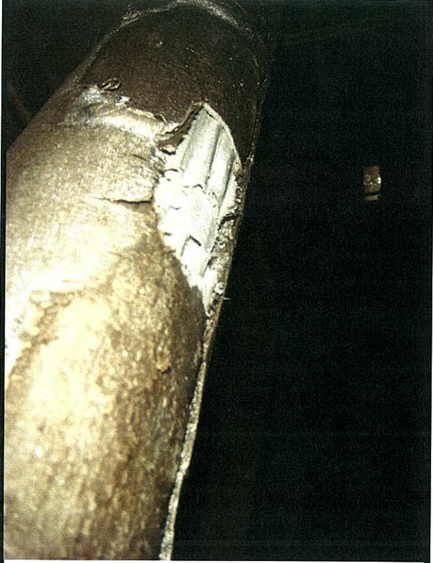
Asbestos Containing Mastic on the bottom layer of floor tile in the kitchen
