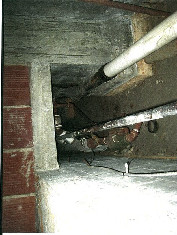
Pipe Insulation on pipes in crawlspace
