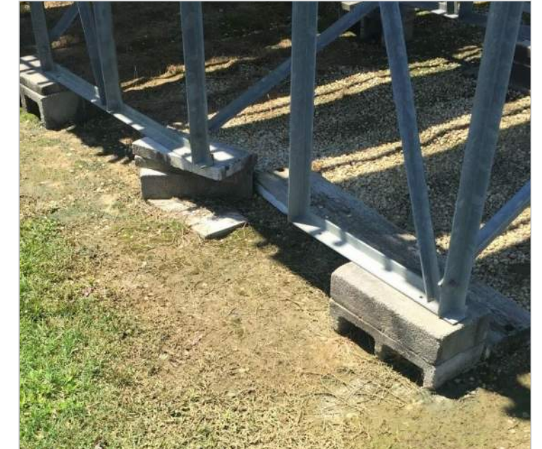
Photo 8: Concrete block support at free-standing bleachers
