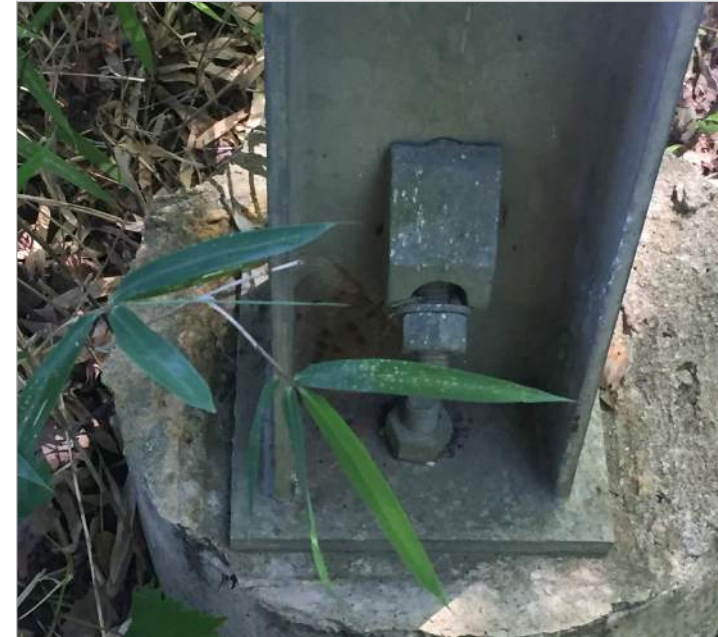
Photo 7: Base of bleacher steel column. No visible rust.
