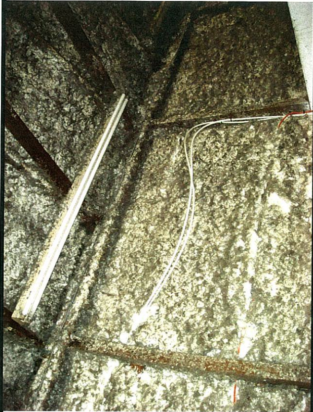
Landfill Maintenance Building Spray Applied Insulation
