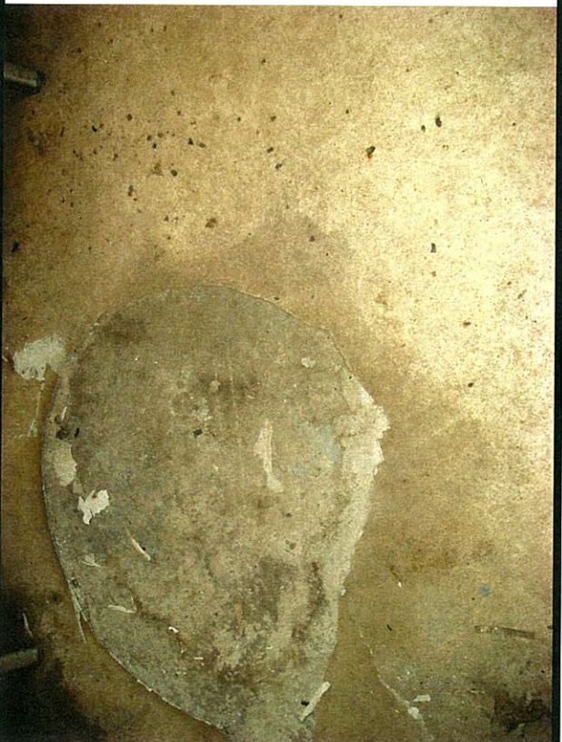
Non Asbestos Vinyl flooring in Office 1
