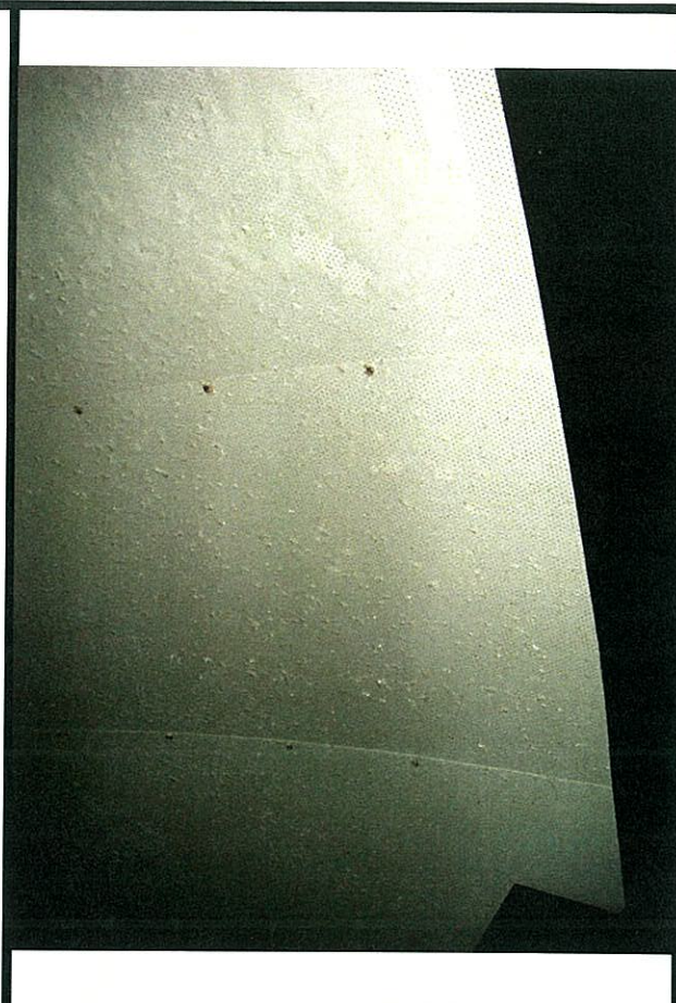
Assumed ACM Roofing material on Entire Building
