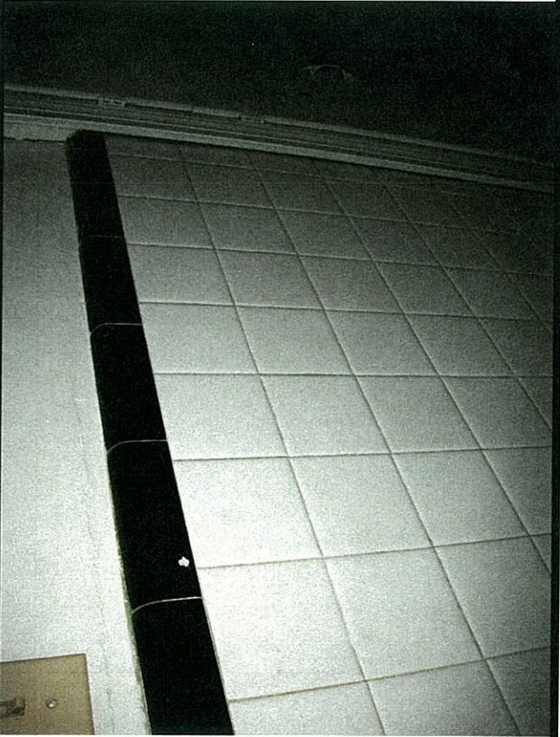
Black Ceramic Tiles Located in Bathroom
