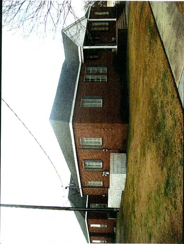
Resource Development Building with assumed asbestos containing roof shingles and window caulking
