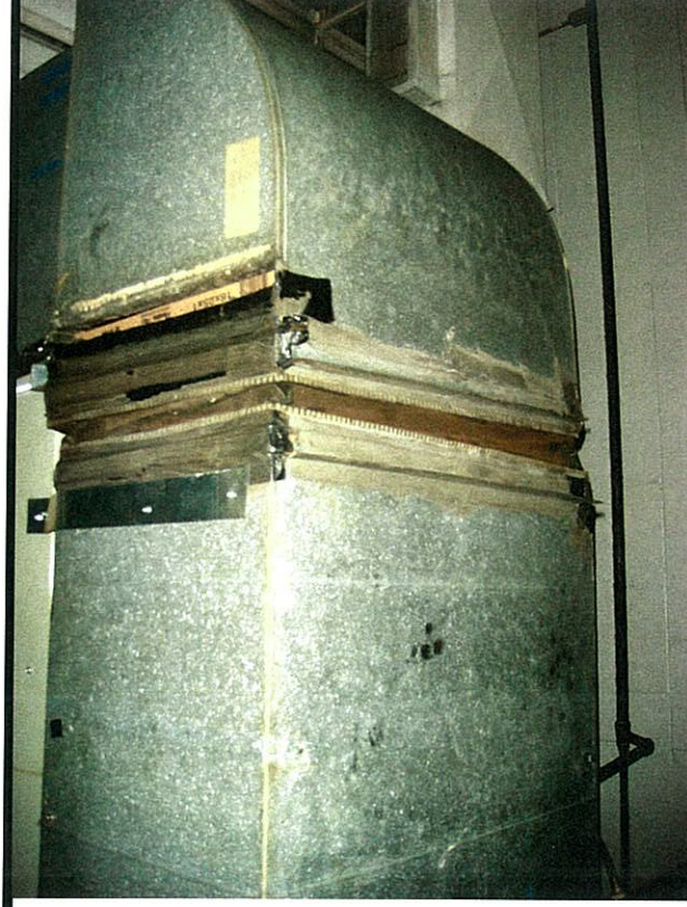
Example of Assumed Asbestos containing Vibration Damper
