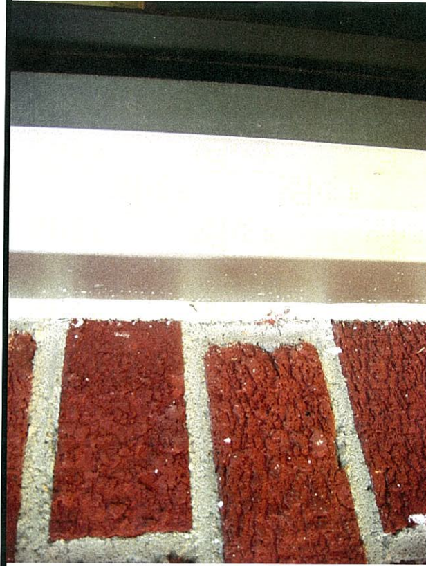
Asbestos containing door Caulking
