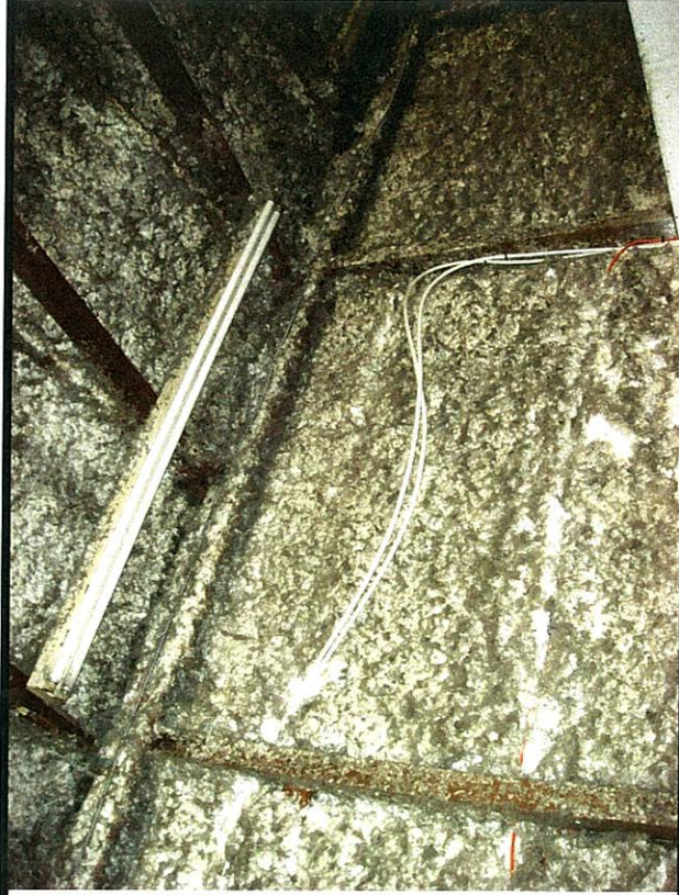
Landfill Maintenance Building Spray Applied Insulation
