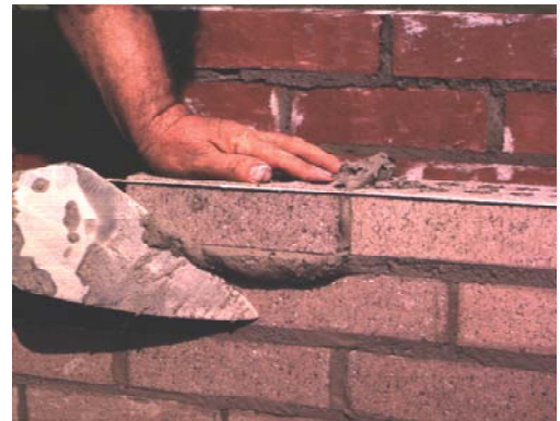
Photo 2 Cutting Excess Mortar
