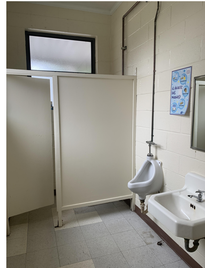
#6: MENS BATHROOM AT LOBBY
