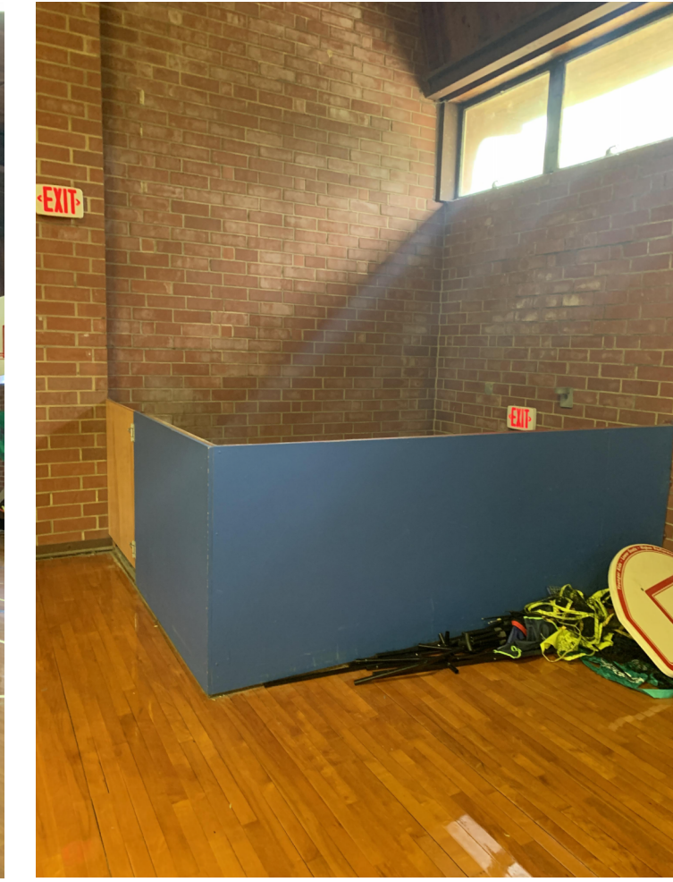
#8: BASEMENT STAIRS AT GYM EAST END
