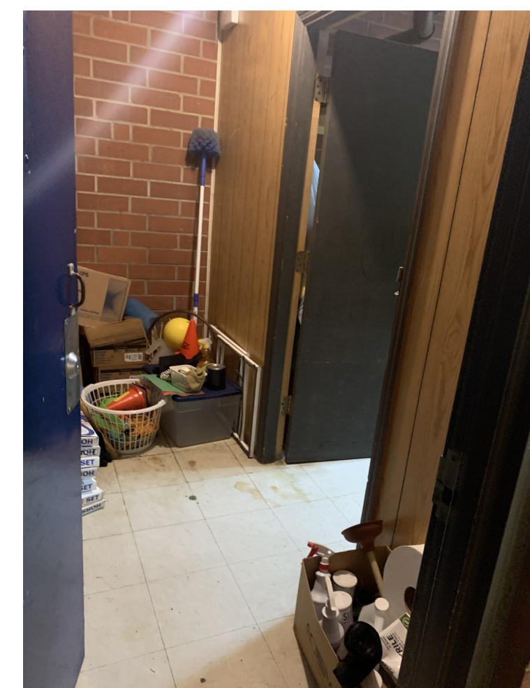
#12: LOBBY UTILITY ROOM
