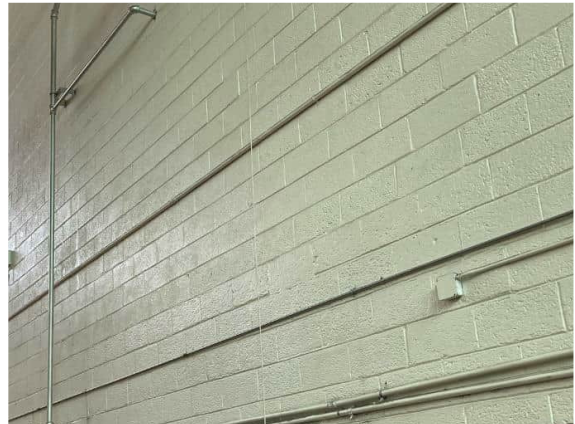
Photo #30 Non-asbestos CMU block coating (HA #33)
