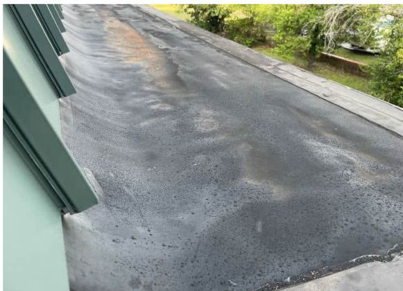
Photo #3 Non-asbestos roofing under rubber membrane roof (HA #3)
