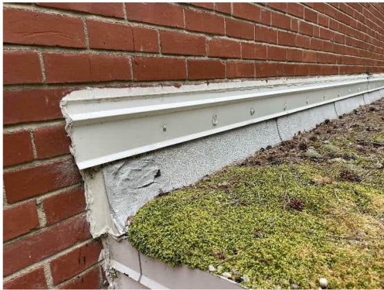
Photo #29 Non-asbestos roof flashing (HA #31) and non-asbestos tan roof caulk (HA #32)
