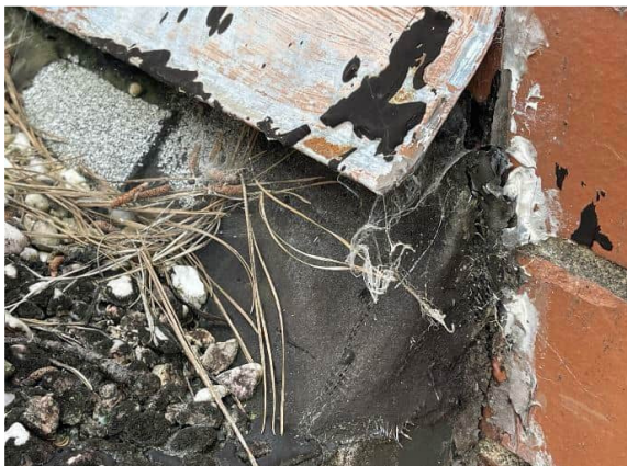
Photo #5 Non-asbestos roof flashing (HA #5)
