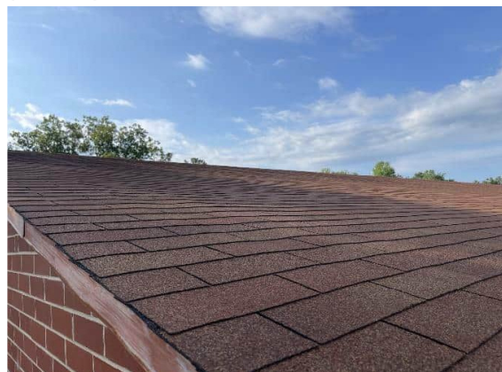
Photo #4 Non-asbestos asphalt-roof shingles/tar paper (HA #4)
