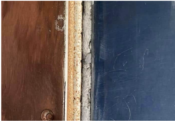
Photo #7 Non-asbestos gray window glazing (HA #7)
