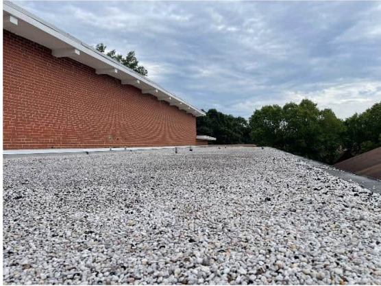
Photo #23 Non-asbestos built-up roofing (HA #24)
