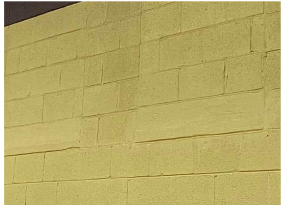
Photo #20 Non-asbestos CMU block coating (HA #22)
