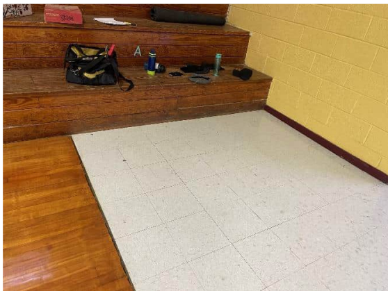
Photo #21 Non-asbestos 12" x 12" light gray floor tile with asbestos-containing mastic (HA #23)
