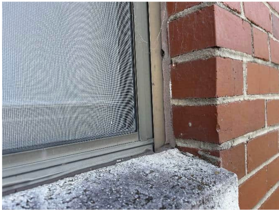
Photo #19 Non-asbestos gray window caulk (HA #21)
