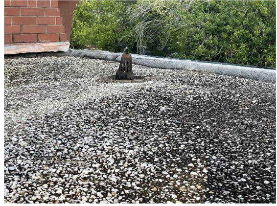
Photo #2 Non-asbestos built-up roofing (HA #2)
