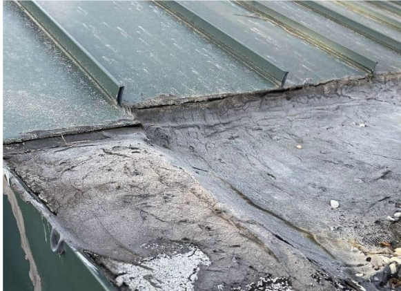
Photo #1 Non-asbestos gray roof mastic (HA #1)
