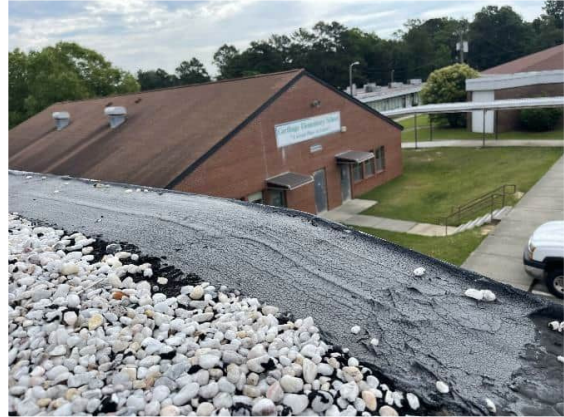
Photo #24 Non-asbestos gray roof mastic (HA #25)
