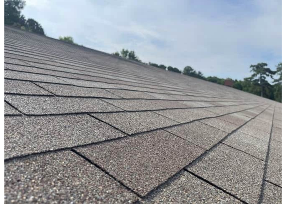
Photo #14 Non-asbestos asphalt roof shingles/tar paper (HA #13)
