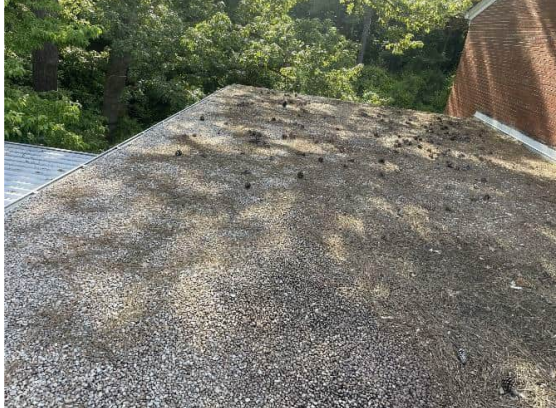
Photo #13 Non-asbestos built-up roofing (HA #12)
