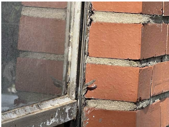
Photo #15 Non-asbestos gray window caulk (HA #14) and non-asbestos white window glazing (HA #15)
