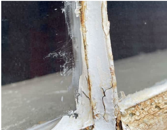
Photo #31 Non-asbestos interior window glazing (HA #34)
