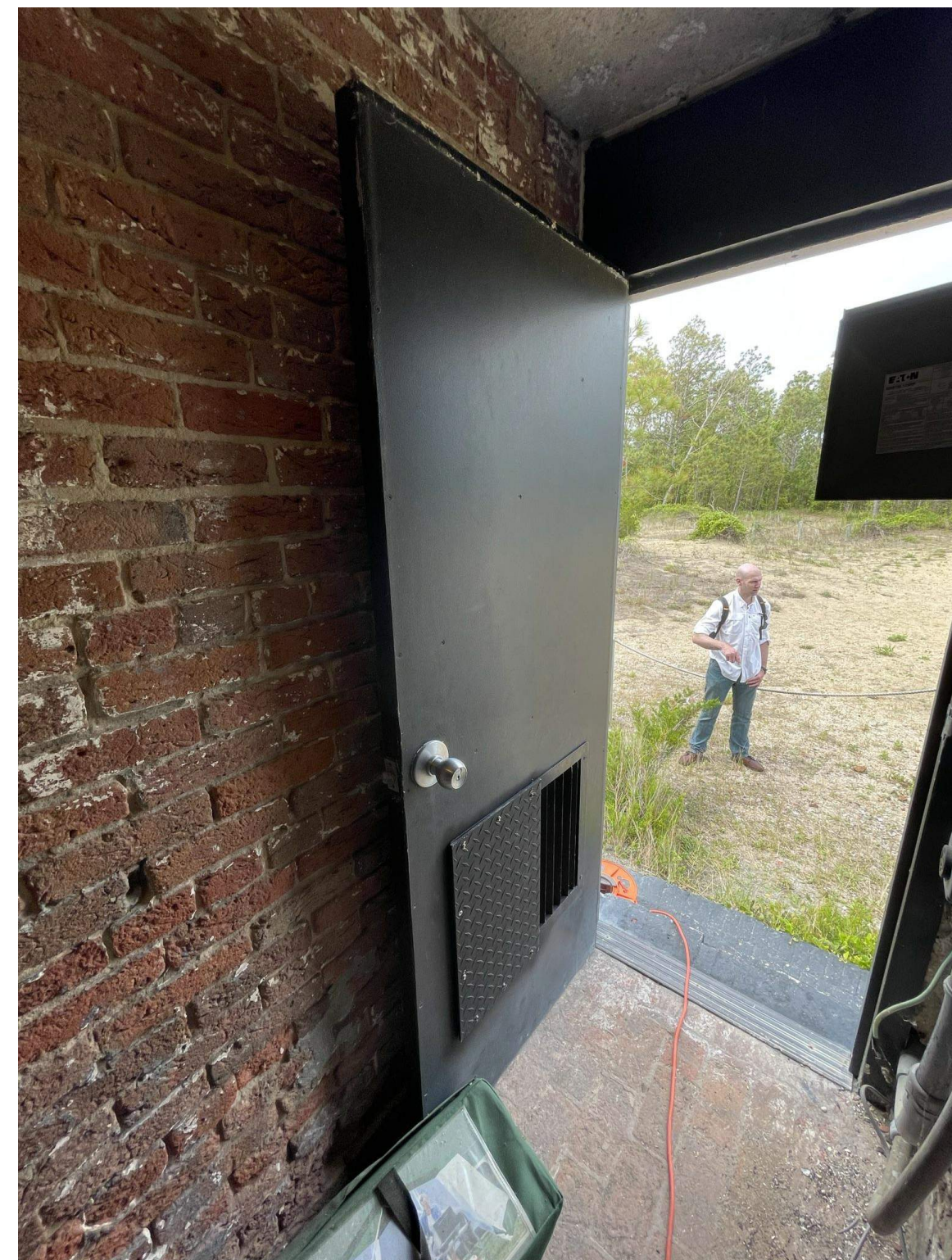
LOWER LEVEL DOOR - EXISTING CONDITIONS
