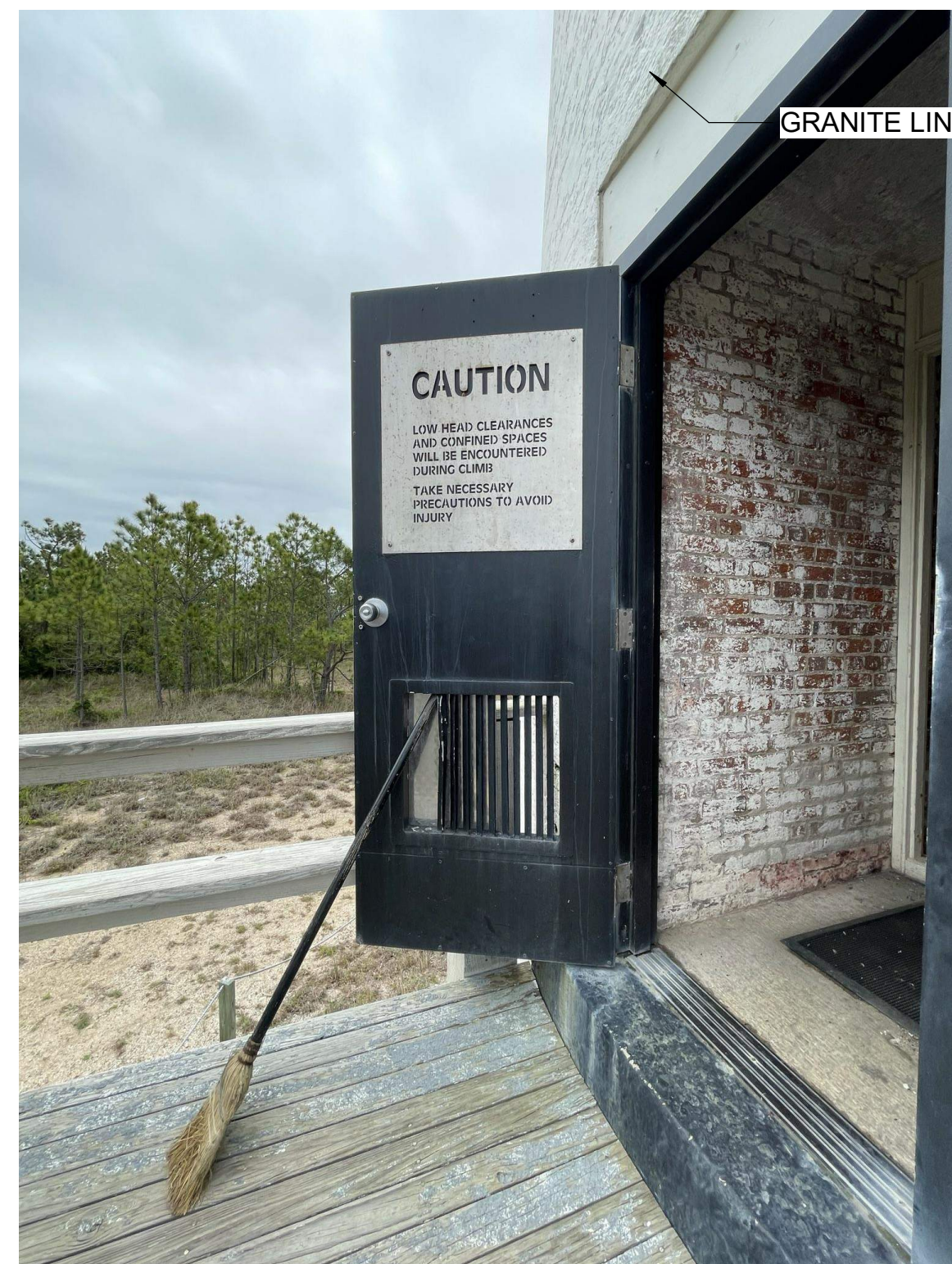
1ST LEVEL DOOR - EXISTING CONDITIONS
