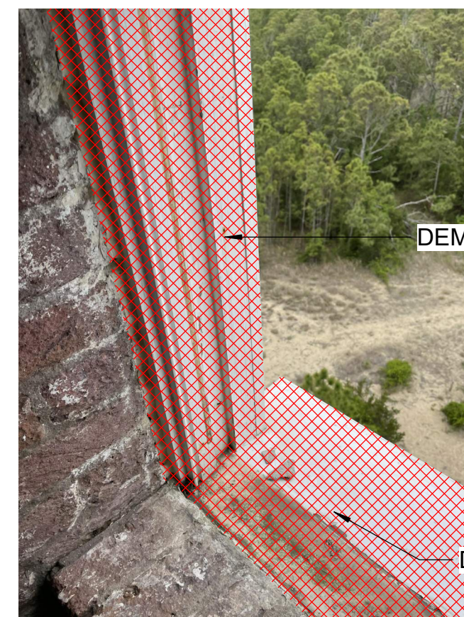
1 TYP WINDOW SECTION - DEMOLITION SCALE: 1 1/2" = 1'-0"
