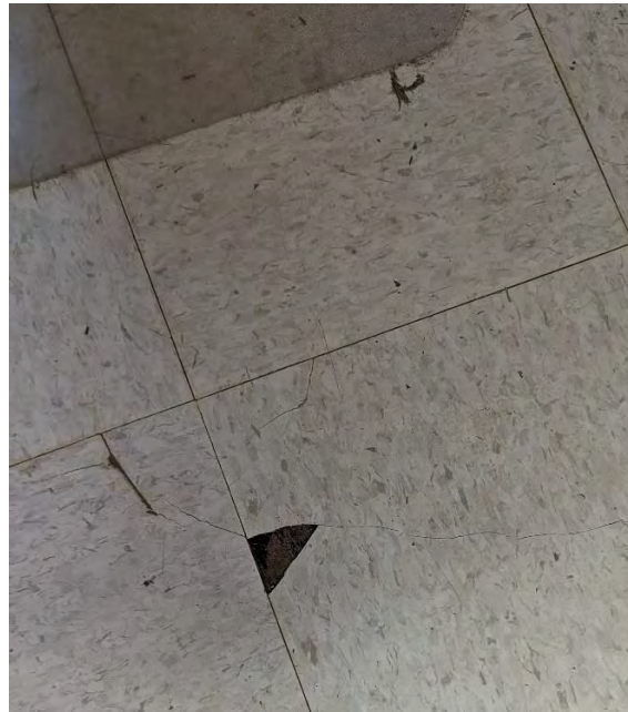
12" Cream W/ Blue Streaks Floor Tile and Asbestos Containing Black Mastic
