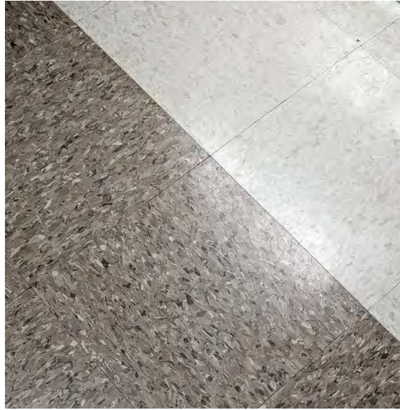
12" Beige Mottled Floor Tile and Asbestos Containing Black Mastic
