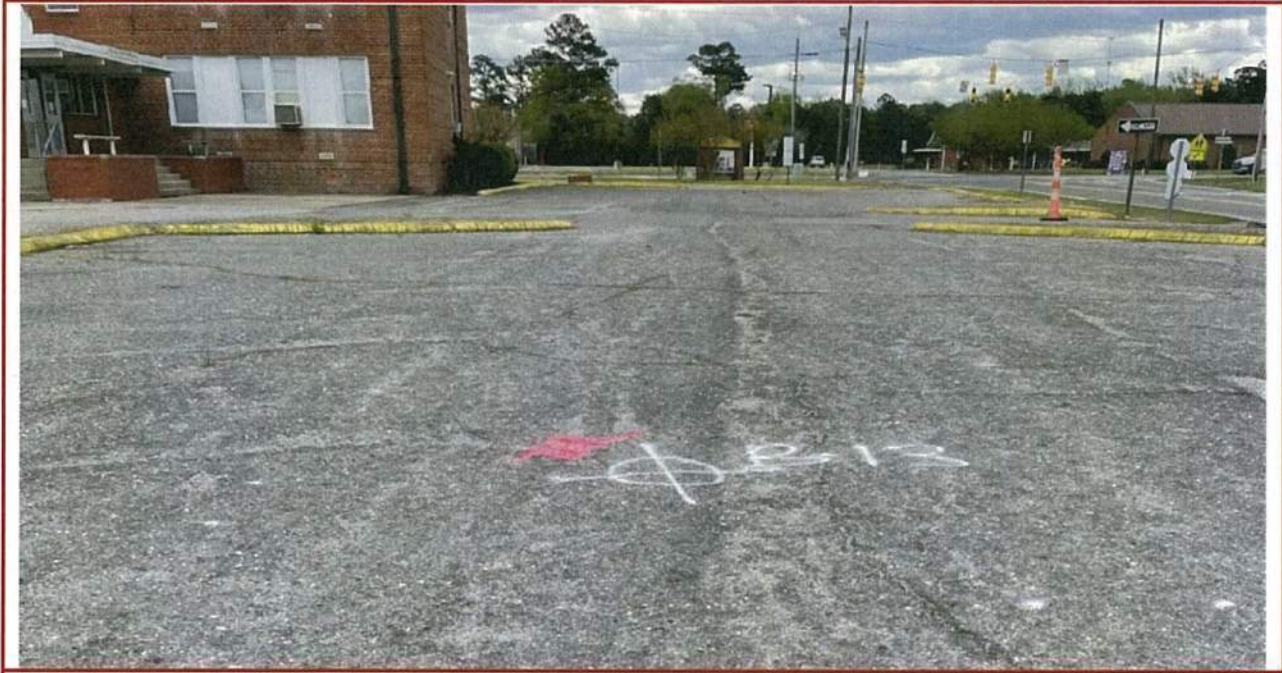
Location B-13 viewing southeast on April 4, 2024
