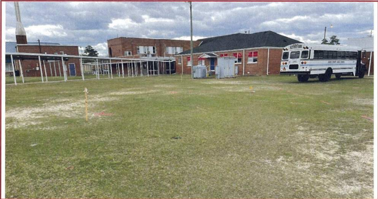
Location B-04 viewing southeast on April 4, 2024
