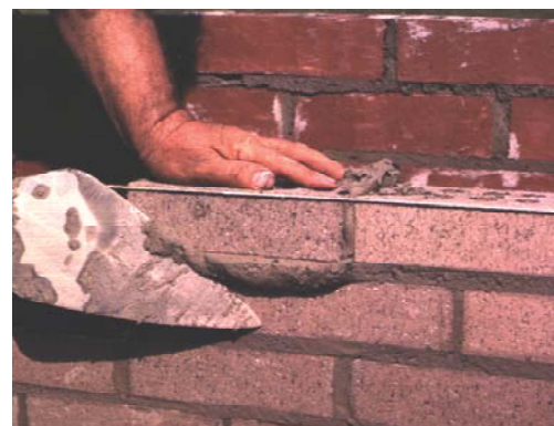
Photo 2 Cutting Excess Mortar
