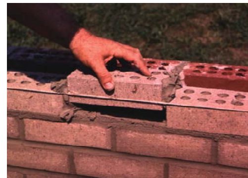
Photo 3 Placing the Closure
