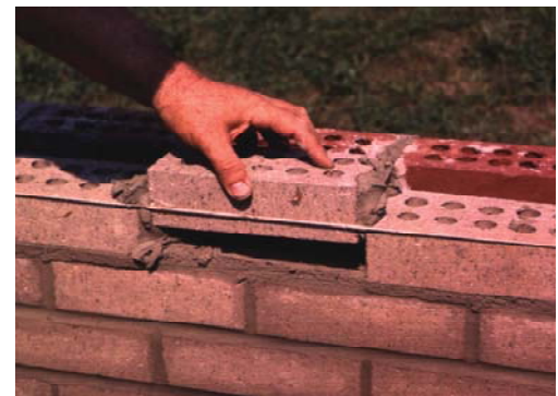
Photo 3 Placing the Closure
