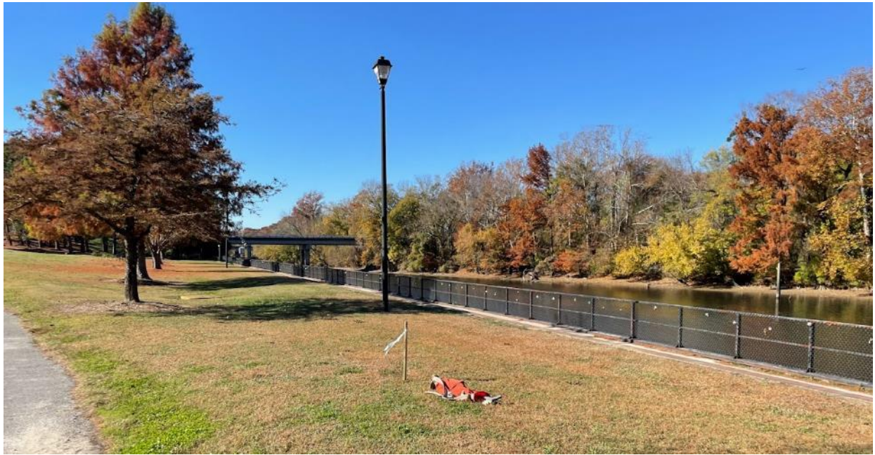
View of the bulkhead facing west
