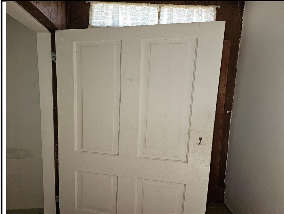
8. Bathroom 3 White Side of the Door
