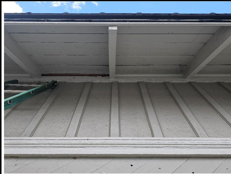
15. White Exterior Frieze Board and Roof Support
