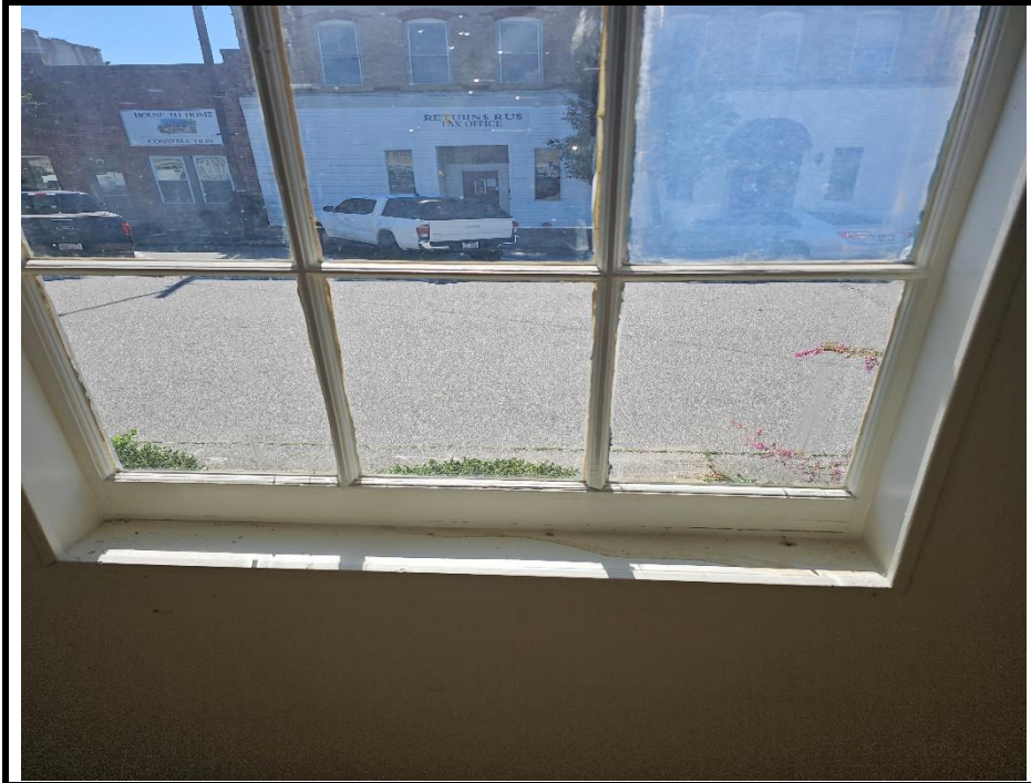
4. Room 5 Window Sash
