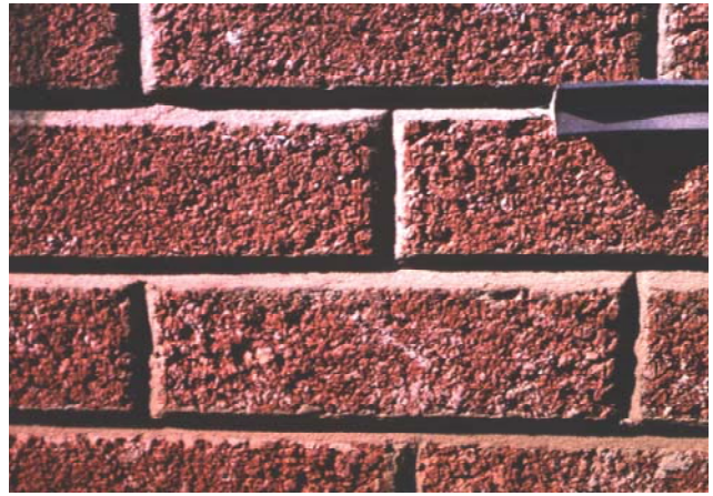
Photo 5 "V" Mortar Joints
